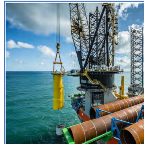
TP lift at Sandbank OWF (GER)
